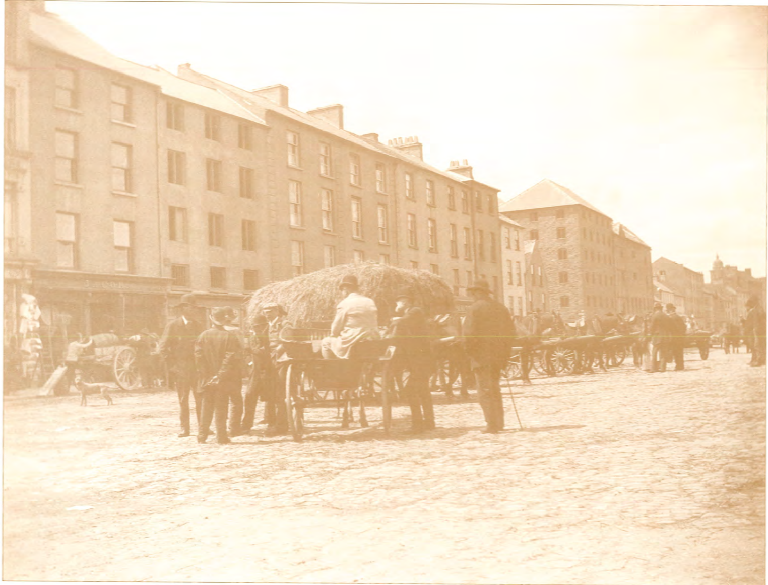
The Granary building (right) on the junction of Merchant's Quay and Hanover Street – about 1900 (Waterford Archive)
