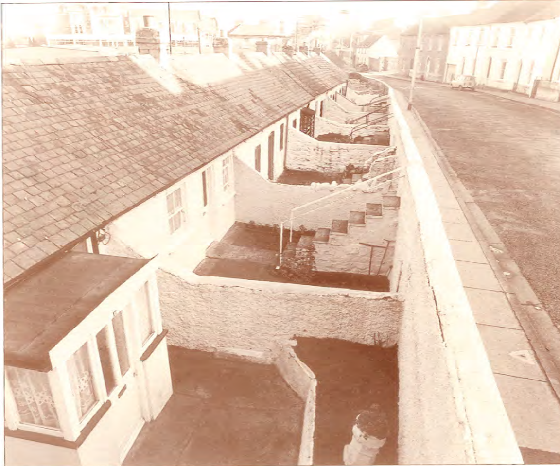
Lower Newtown 1977. The row of houses known as Bailefoidín was demolished in 1985 (Waterford Archive)
