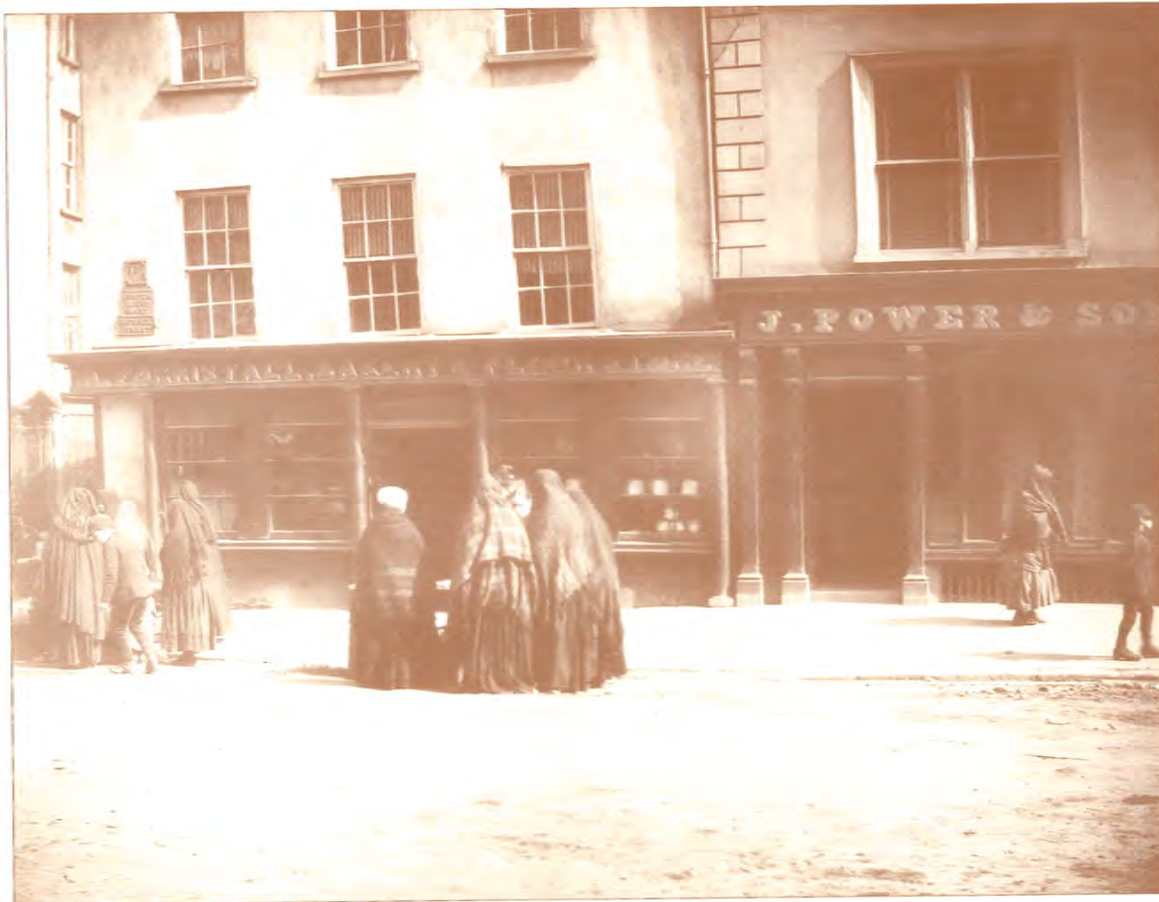
Michael Street. Corner of Peter Street – about 1895 (Waterford Archive)
